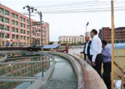
Water Treatment Plant, KEPZ
