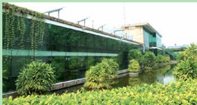
LEED Platinum certified garments factory Vintage Denim Studio Ltd. of Ishwardi EPZ
