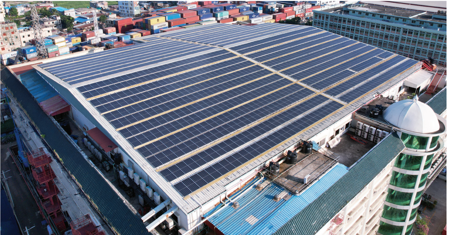
Solar panels cover the entire rooftop of a factory building of Chattogram EPZ
