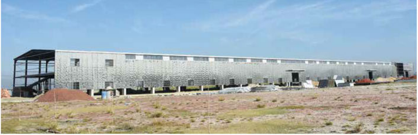
An under construction factory building of BEPZA EZ
