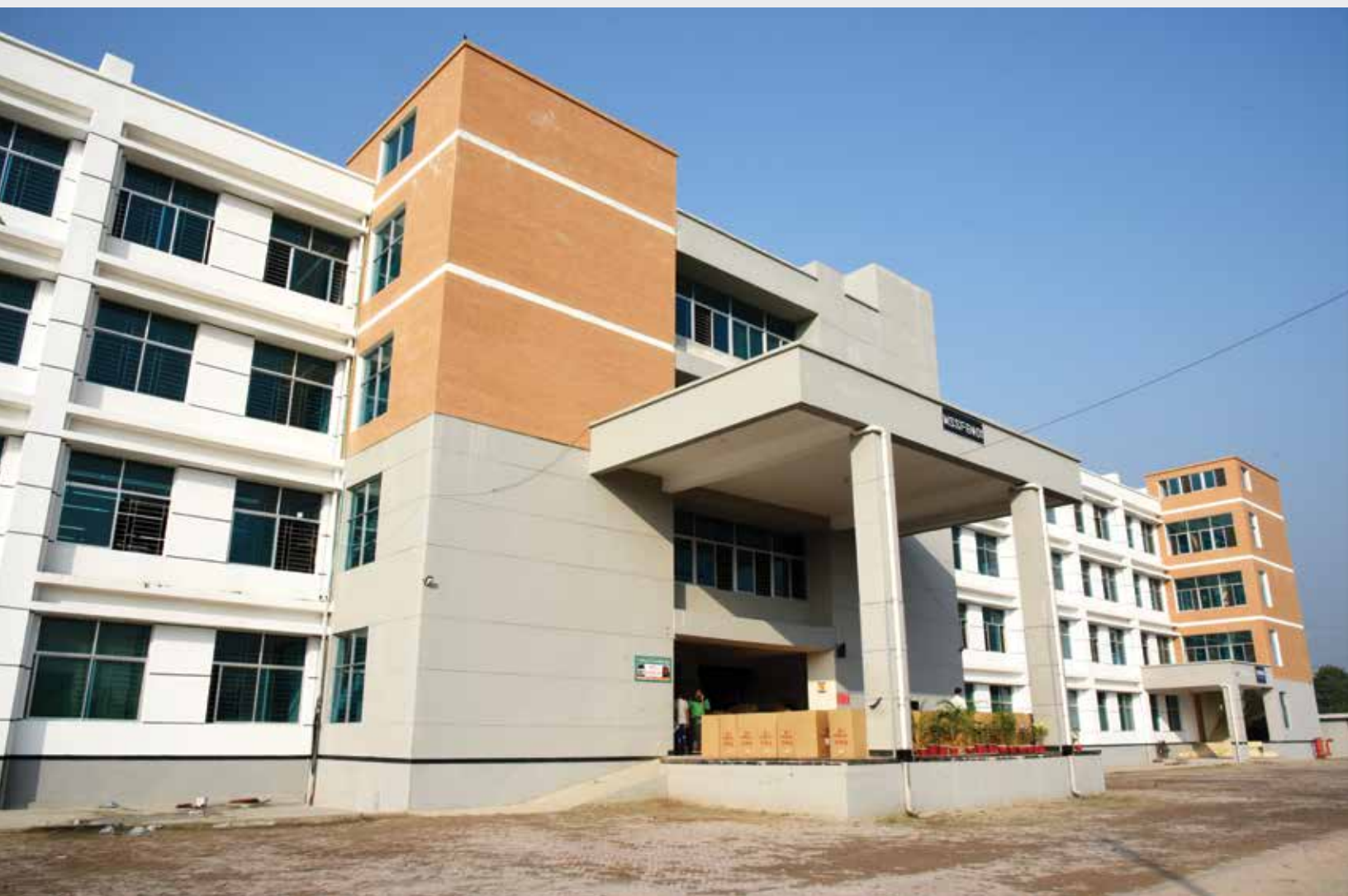
Standard Factory Building of the Zone
